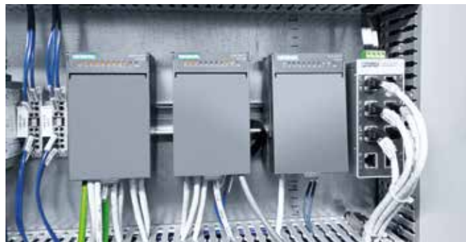
Networking of all devices with PROFINET and Ethernet.
