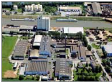
The building at GKN Trier covers 31 000 m 2 .
