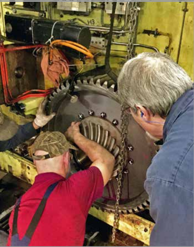
Checking the clearance of the new intermediate gear wheel after reassembly.
